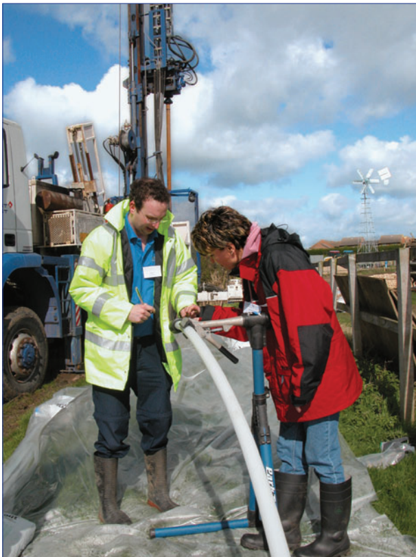
Construction of CMT ports in a 7-Channel system installed in Silsoe, England.
